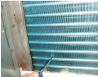
3. Use a flat screw driver to create 1/4" gap between 2 fins (between 2nd tube and 3rd tube) to accept the sensor.
