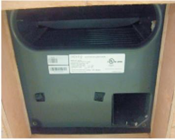
1. Before template installation, with upper unit placed over opening; the freeze sensor should be installed in evaporator coil.
