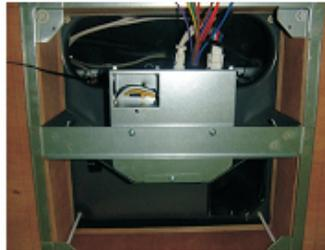
5. Install the template and electrical box on the ceiling.
